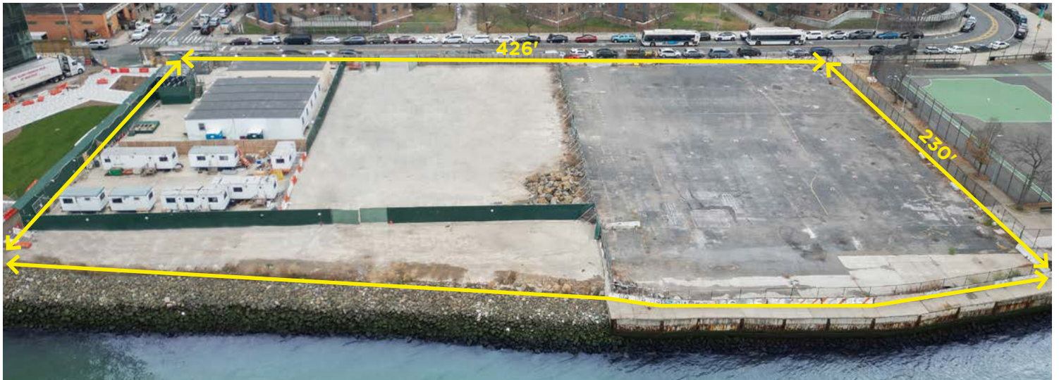
40/50 HALLETTS POINT SITE
